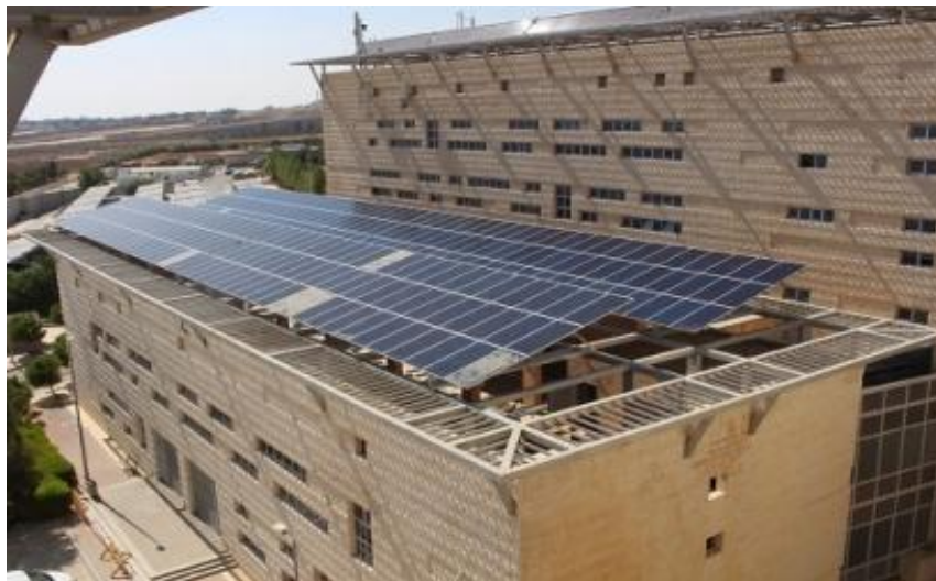
Figure 12: PV system rooftop installation.
