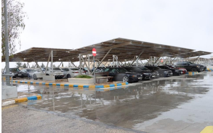
Figure 13: PV car park.
