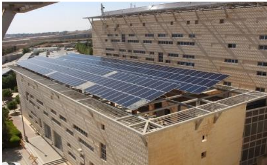
Figure 12: PV system rooftop installation.
