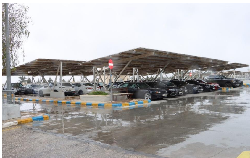
Figure 13: PV car park.
