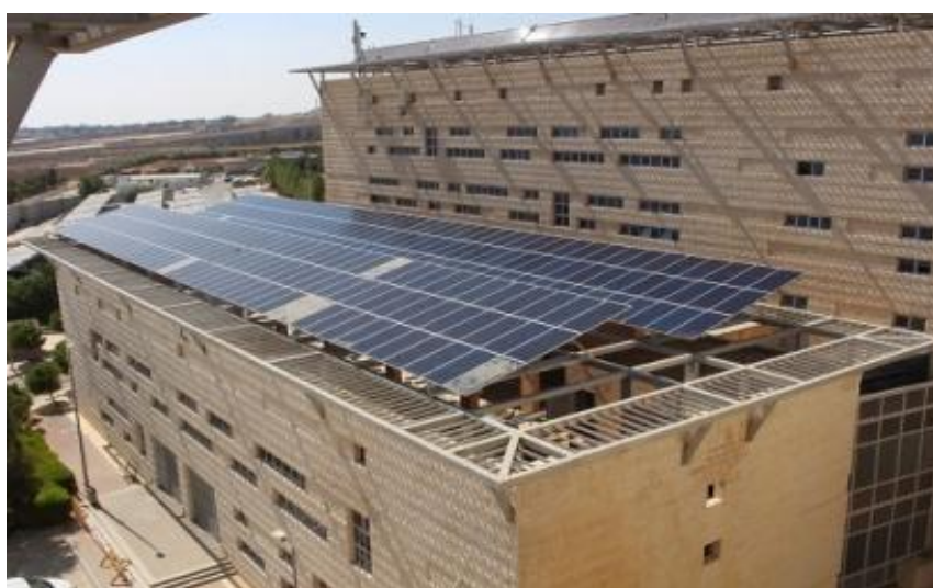
Figure 12: PV system rooftop installation.
