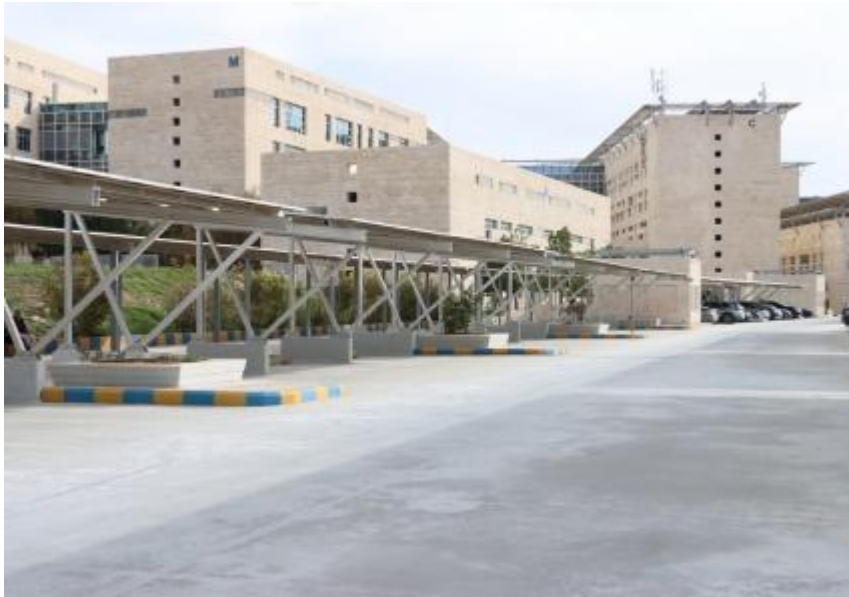
Figure 23: Student parking area.
