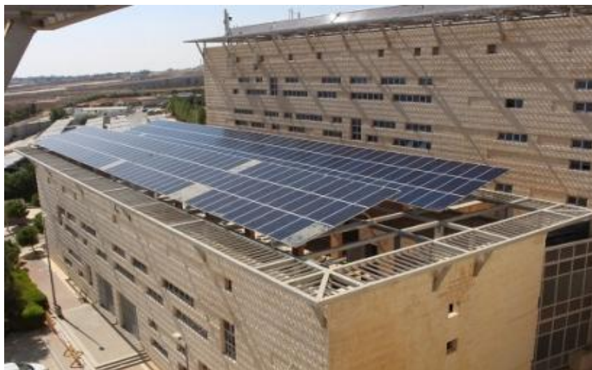
Figure 12: PV system rooftop installation.
